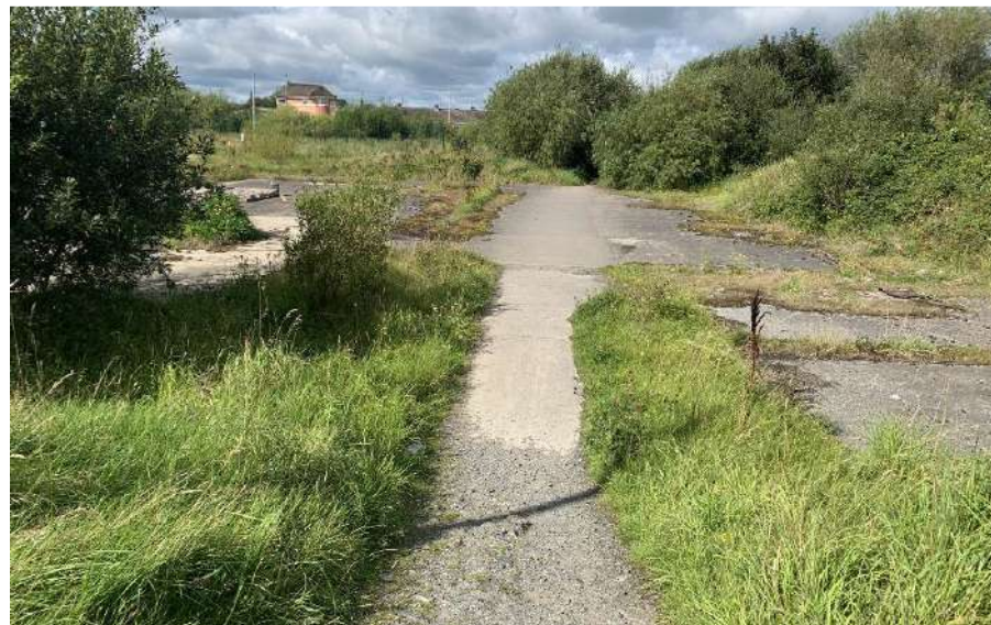
Plate 2: Concrete pad, facing west
